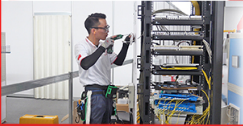
Information Network Cabling
